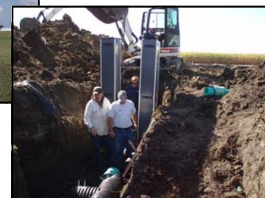
Surge Pond Construction (below)
